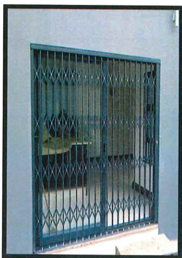
Expandable gate for the sliding door - Burglar bars for the windows – Expandable gate for the front door
